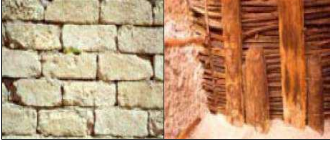
Figure 6. Construction materials (limestone blocks/ palmwood). Source: Ercan Dagli, Philippe Stehlik (2005)
